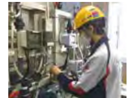
予防保全 Preventive maintenance
